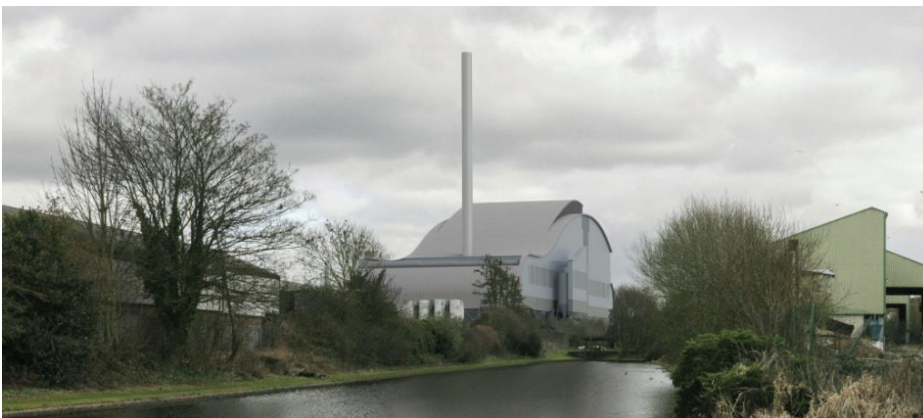
Image courtesy of enfinium.co.uk and GSDA architects
